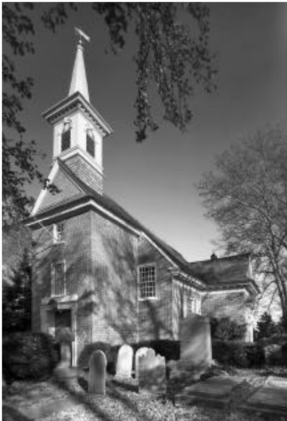
The exterior of Gloria Dei Church after its 1999 restoration.
