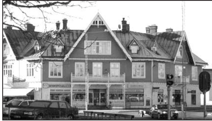
Located in the center of town, Lisselska huset (the Lissel's house) is known today as the most recognized building in Malung.
